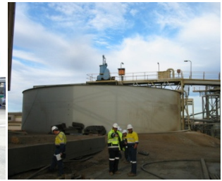
Minesite fuel storage
