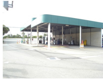
Bus depot fuel storage
