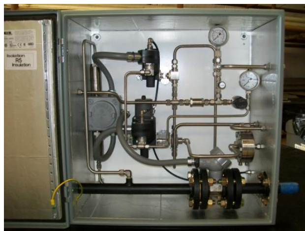
Pic 5. Quick install consolidated valve box 24 x 24 x 12 inches
