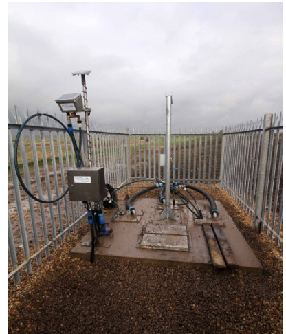
The 3 Airwell pumps installed on site
