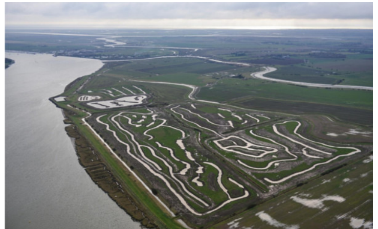
The Lower Raypits Conservation Wetlands
