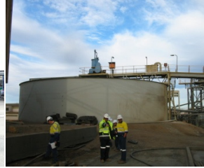
Minesite fuel storage
