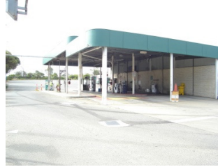
Bus depot fuel storage
