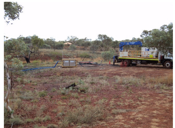
Airwell flow testing skid and truck setup on site
